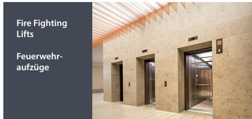
Fire Fighting lifts are designed according to EN 81.72 to be used both as standard lifts and by firefighters during emergencies. In the event of a fire, the firefighter can set the lift to priority mode by turning a key used to command the lift only from inside the car.
